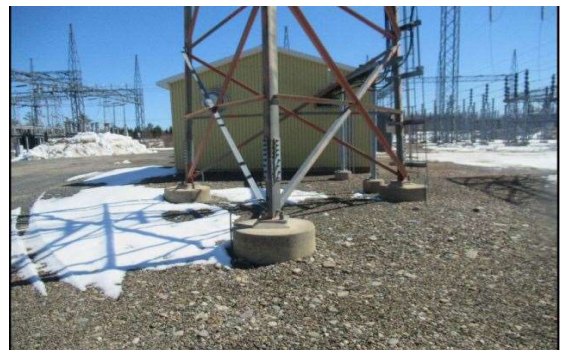
Photo 2: Base of the tower.
