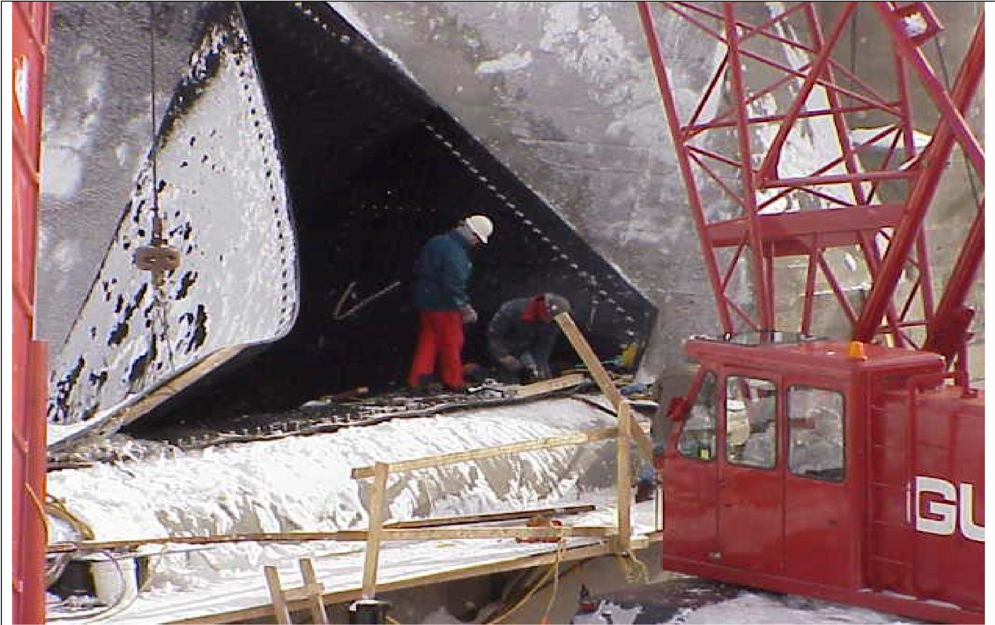
**Final Fitting of the Rubber Dam on the South End of the Main Dam, 1999 6**
