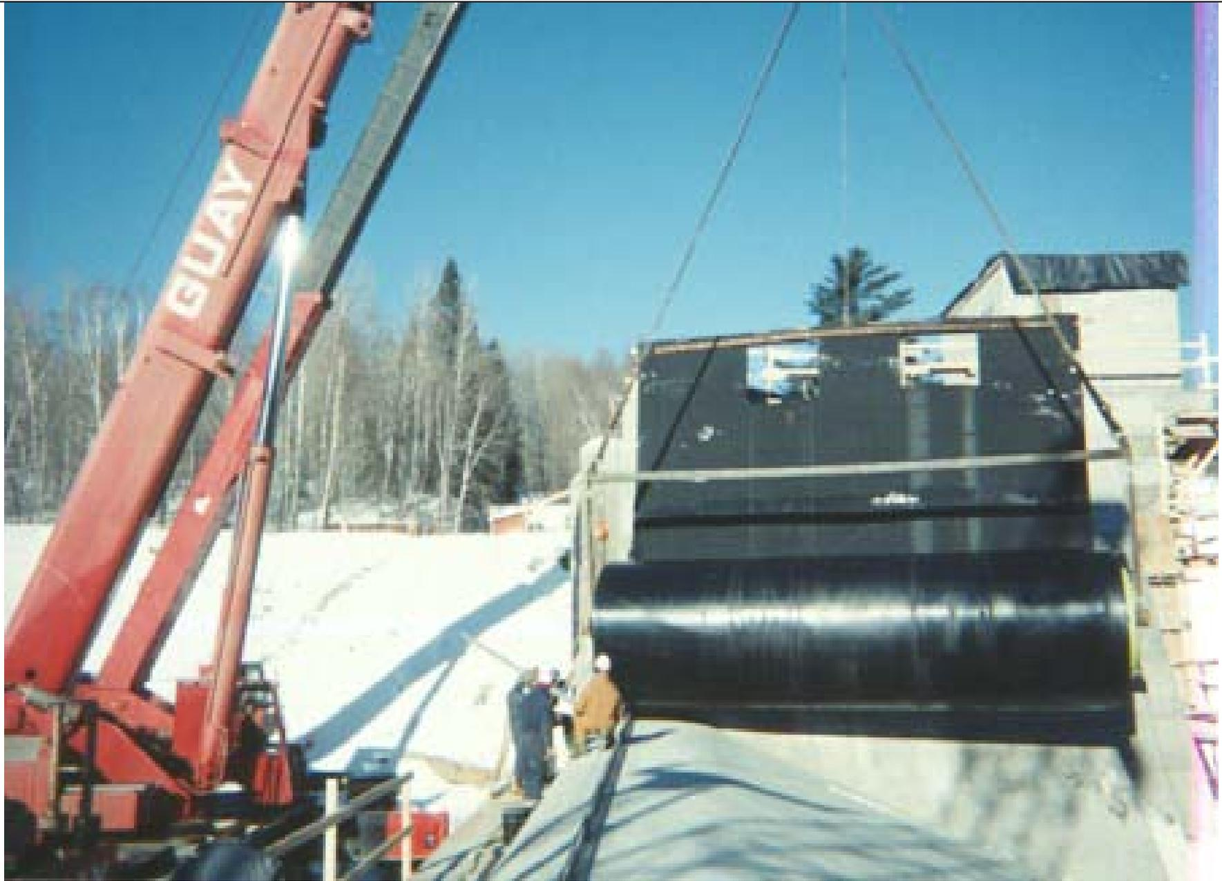
**Rubber Dam being Rolled out on Main Dam, 1999**
