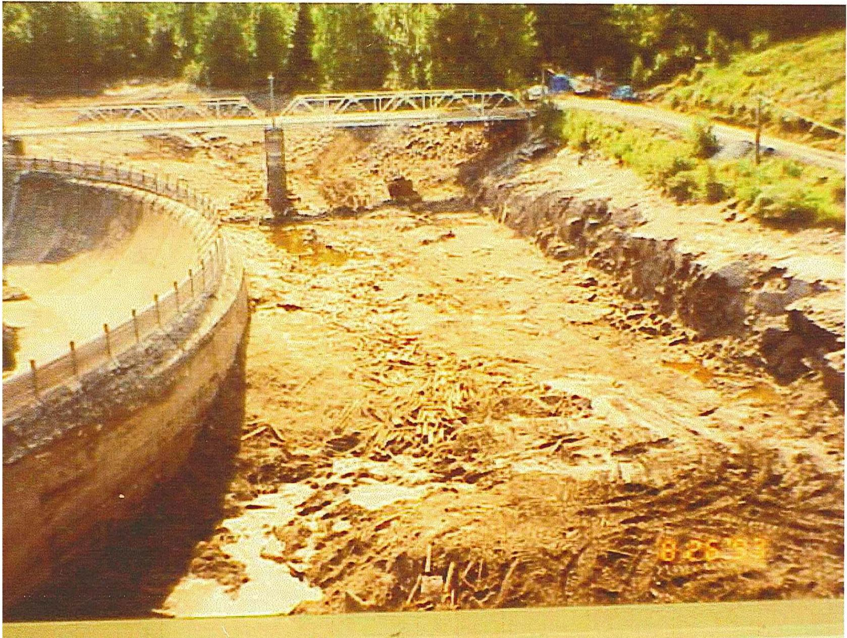
**View of the Spillway Dam Showing Wooden Flashboards and Forebay Flood Dewatered (1993)**
